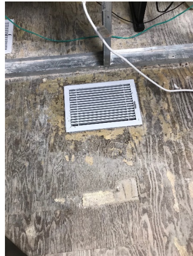
Figure 4: Room 118/GIS Lab Example of Wooden Sub-Floor to be Removed
