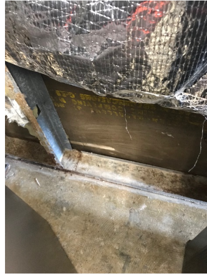
Figure 2: Room 121 Drywall to be Removed
