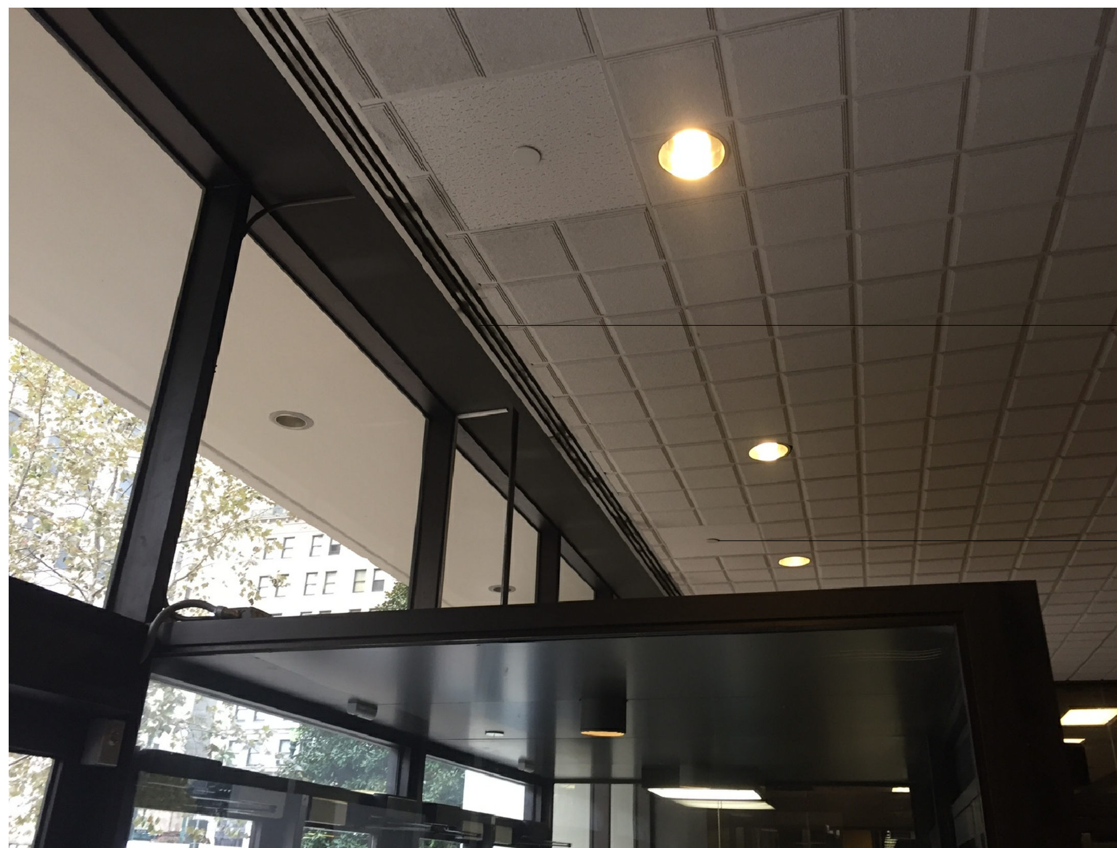
2 EXISTING LOBBY CONDITION NTS
